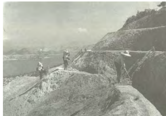
Conservation work; Construct stair cutout
