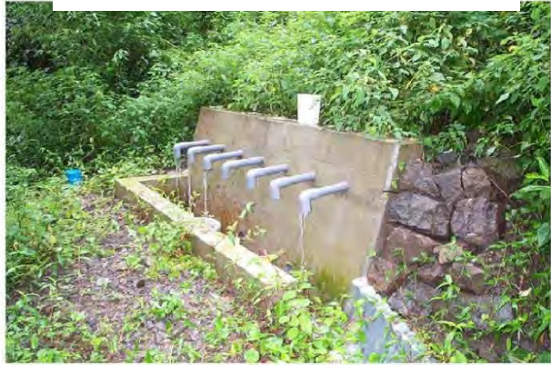
Drainage drilling work
