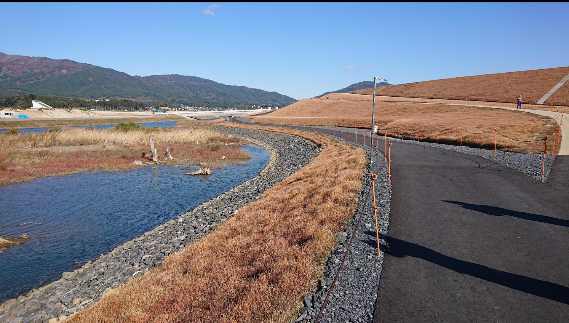
防潮堤の陸側は覆土・緑化され、湿地が保全された The seawall was covered by grass, and wetland was conserved.
